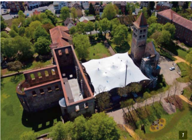
Figure 1: Convertible roof of the open-air theatre in Bad Hersfeld 1968 (replaced in 2019).
